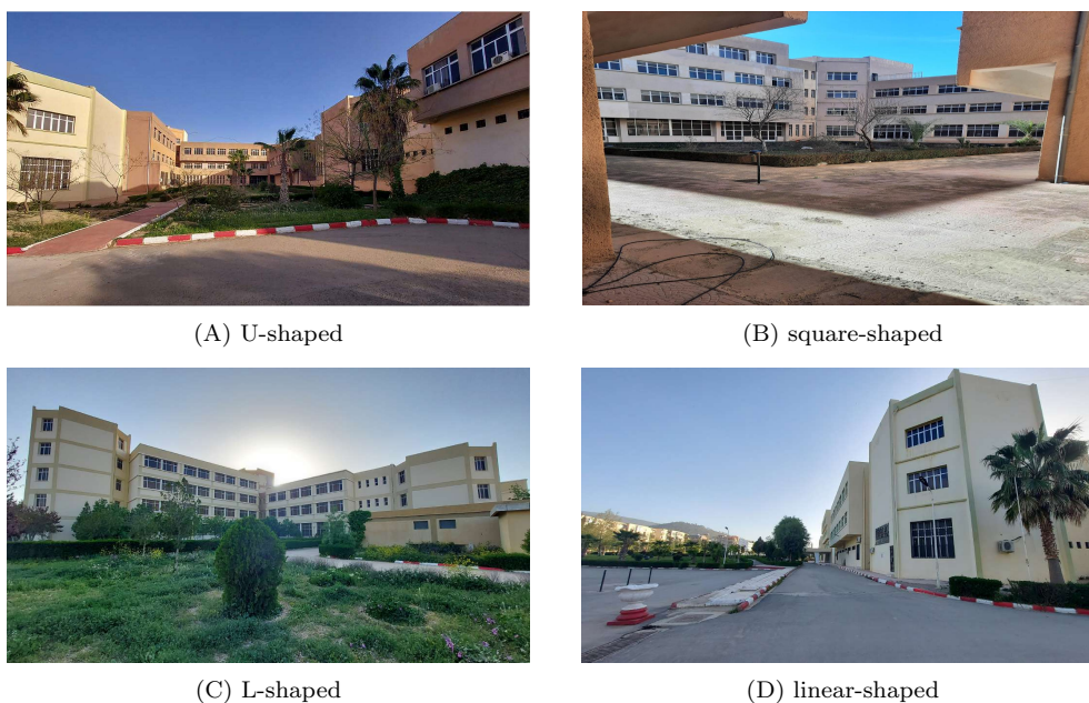
FIG. 2. Photographs of each measurement stations.
