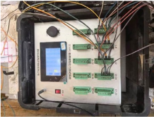
(b) Stress monitoring system
