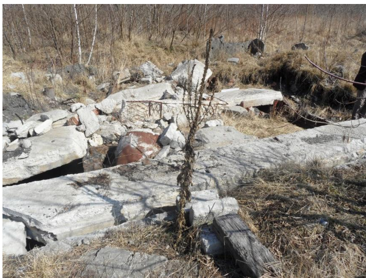
Fig. 4. View of the destroyed shaft capping slab P
