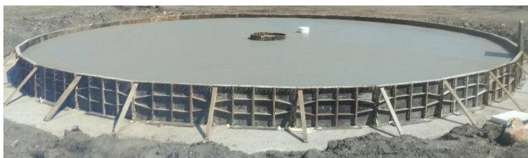
Fig. 12. View of the concrete slab
