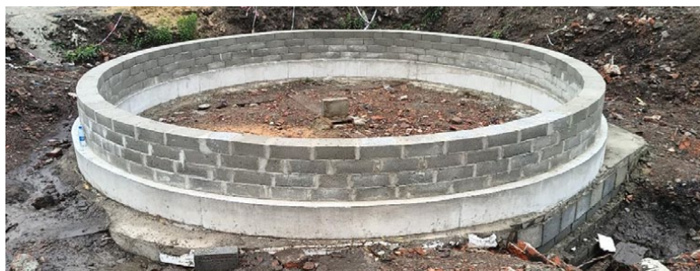
Fig. 10. Reconstructed masonry lining fragment at the shaft collar
