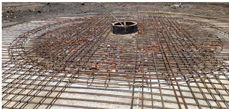
Fig. 11. Reinforcement of the slab sealing the shaft
