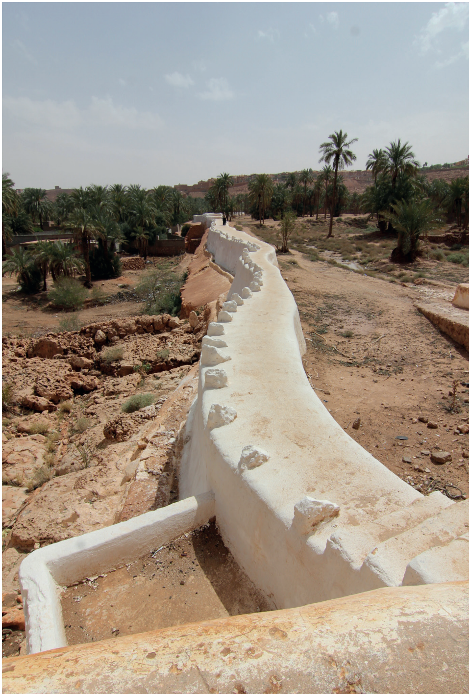
Figure 4. The passageway of Beni-Isguen dam (A. Kasmi)
