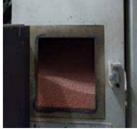
Fig. 13. Uncontrolled Waste Powder Container
